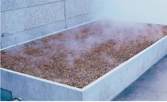
Fig. 2.50 Biofilters have been extremely successful in reducing odor emissions in a natural way.
