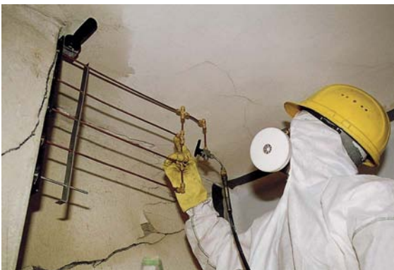
Fig. 3.114 Gelatine is a proven agent for decontaminating buildings containing asbestos.
